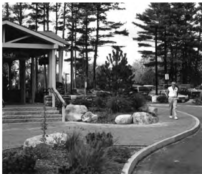
Granite curbing holds up well to snowplows and heavy traffic while providing a solid edge for sidewalk paving.
