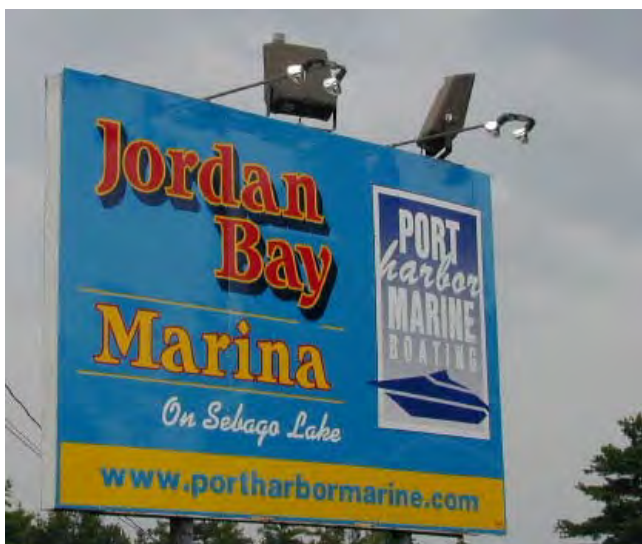
These top-mounted light fixtures are not well shielded nor integrated into the sign.
