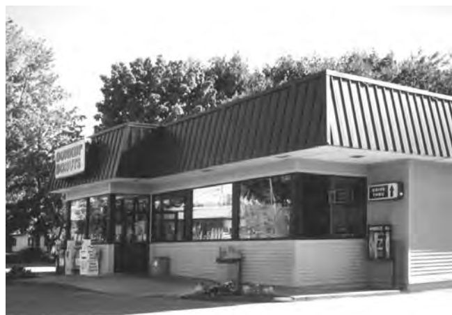
The use of false mansard roofs or vertical panels are inappropriate for rooflines.
