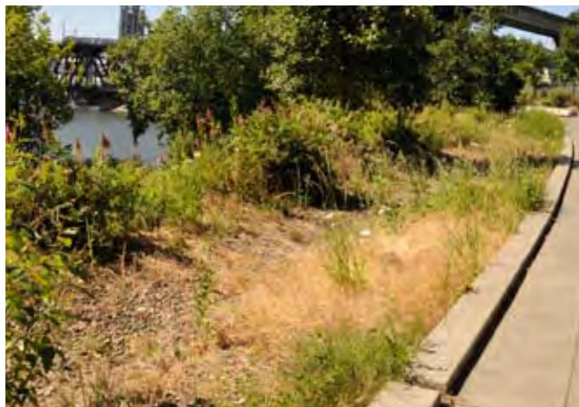
A vegetated swale next to a walkway absorbs runoff from the paved surface and filters stormwater.
