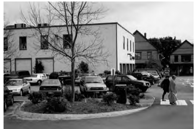
A raised walkway through this parking lot provides a safe, attractive pedestrian route. Reflective paint used in the crosswalk marks the route in a highly visible manner.
