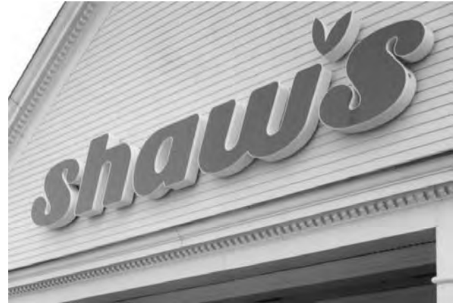
An effective use of individual internally-lit letters to create a simple identity for a commercial building.
