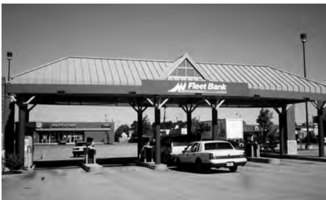
By using the same form and materials the canopy over the drive-through is visually compatible with the main bank building.
