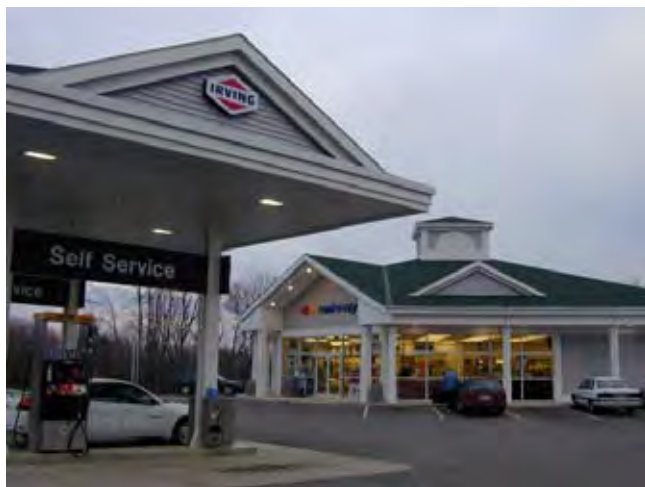
The gas station canopy has been designed to complement the main building. The town strongly encourages the use of attached canopies, especially in service stations that are being retrofitted.
