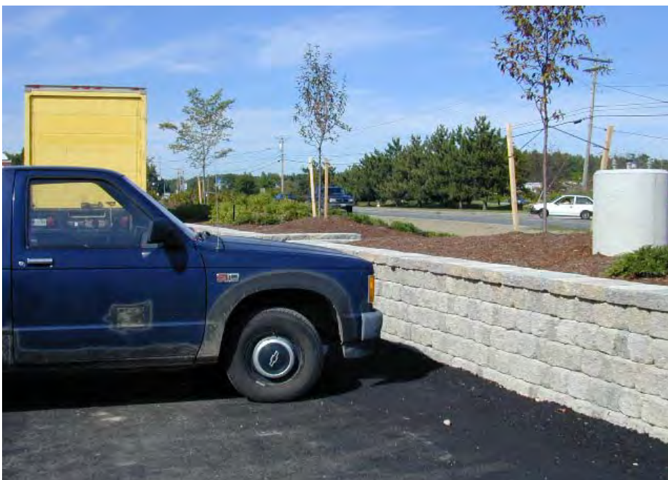
Parked cars are effectively screened by a low concrete block wall and ornamental plantings.
