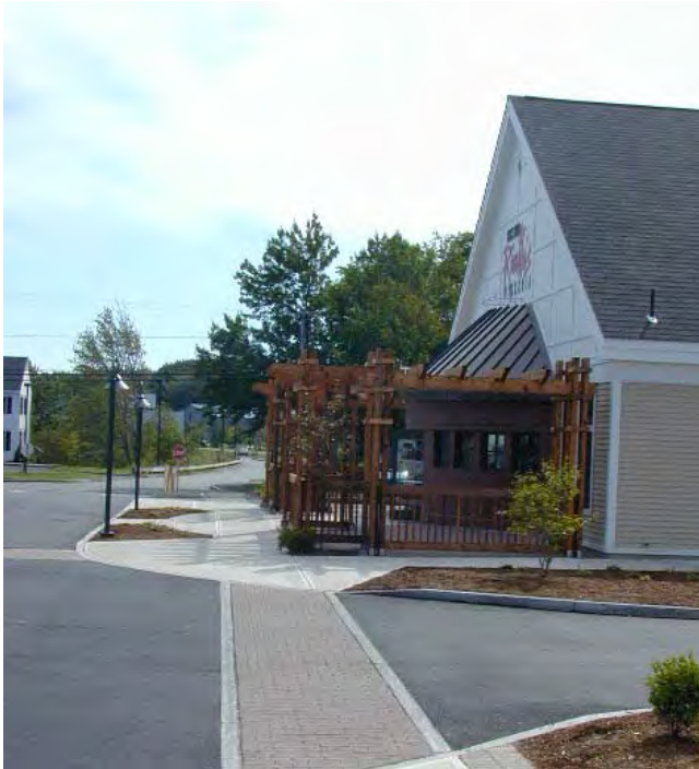
Concrete pavers create a permanent crosswalk that affords good visibility and contrasting surface texture.
