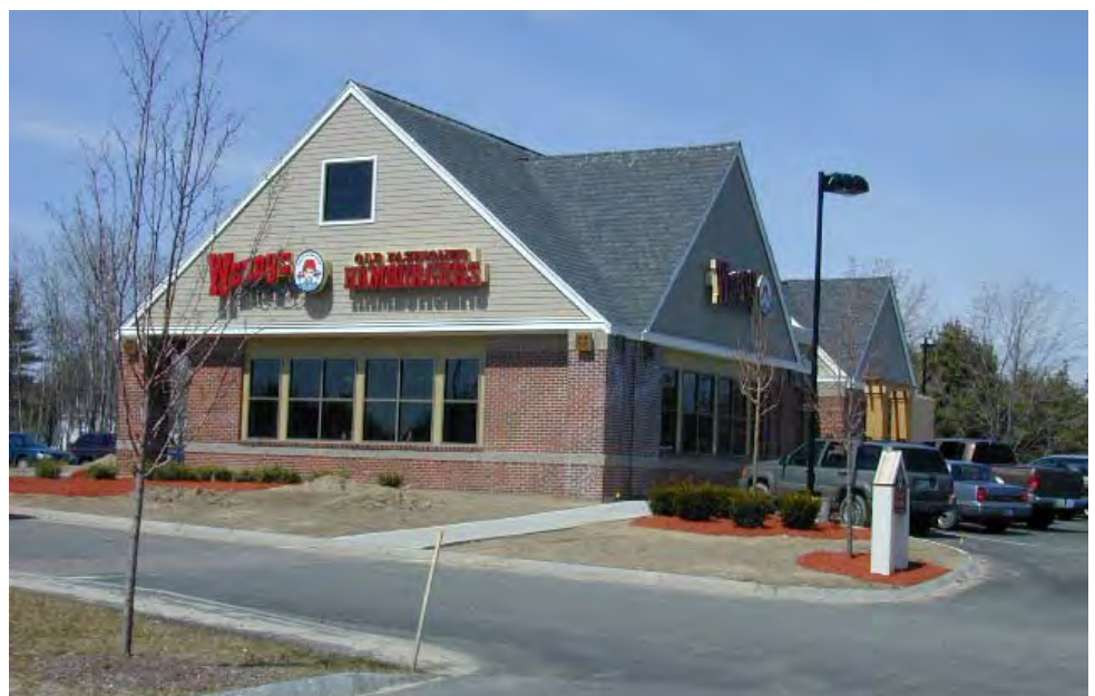
A restaurant that was designed to complement the vision for a highway corridor.
