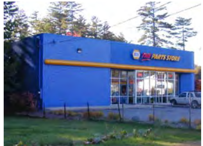
Highly reflective surfaces and bright colors are not characteristic of traditional New England architecture.
