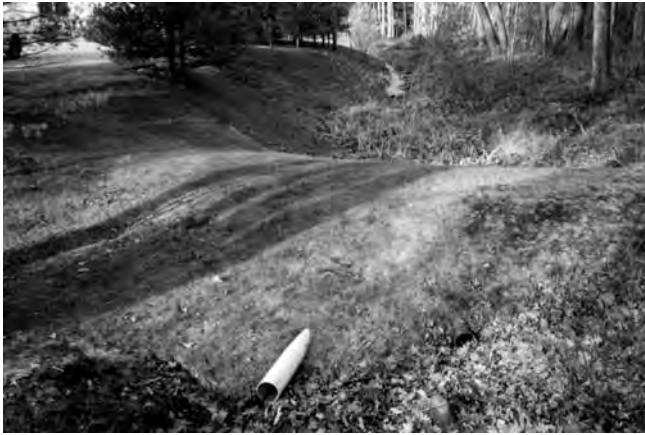
This stormwater management facility has been designed to blend into the landscape through transitional grading. The outfall pipe should have been integrated into the design.
