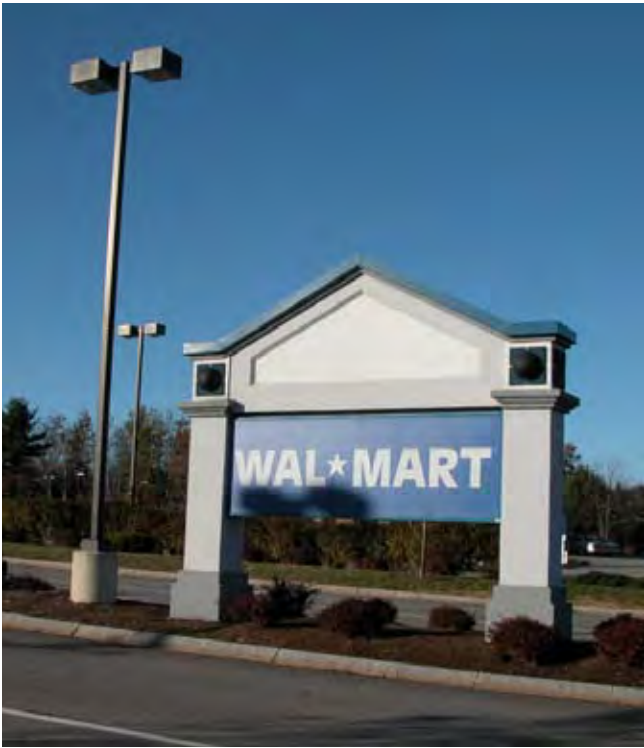
Simple 'shoe-box' fixtures mounted on square poles provide a clean look that complements the site.
