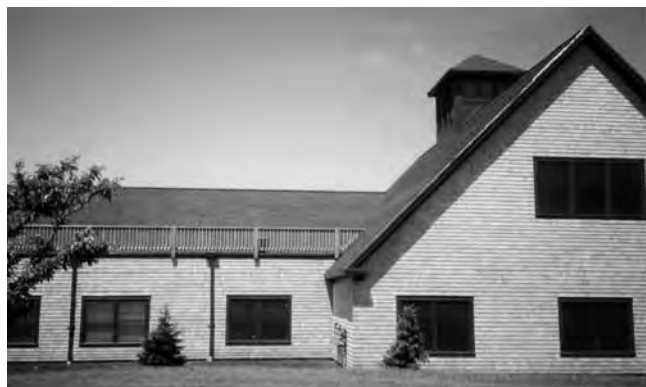
Roof-mounted mechanical equipment has been effectively screened by balustrades.
