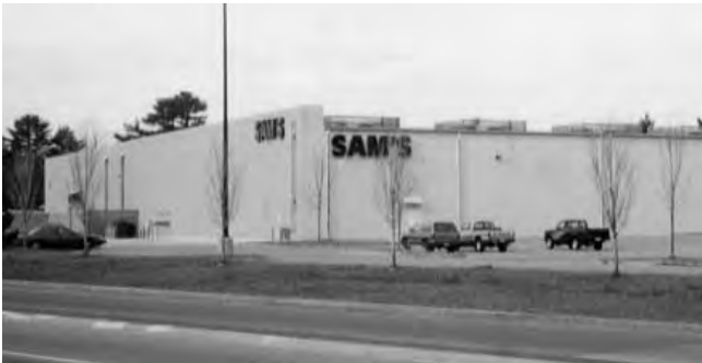
Painted concrete block
