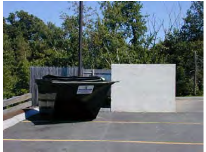
This trash enclosure was not properly sized to handle the dumpster needed for the facility.
