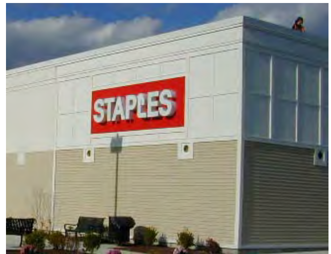
This sign is well integrated into the design of the side facade, displaying only the essential information.
