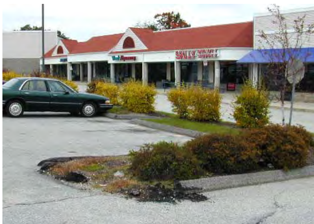
While asphalt curbing is inexpensive to install, it is very prone to snowplow damage.
