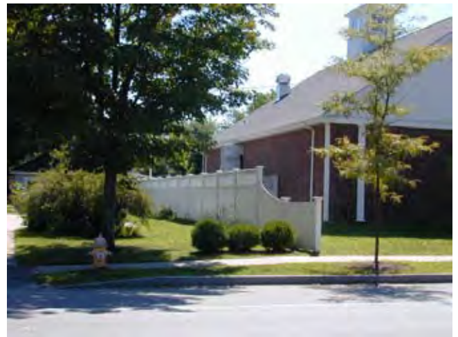
A variable height fence used to provide visual separation between a convenience store and its residential neighbor. Note exterior storage behind fencing.
