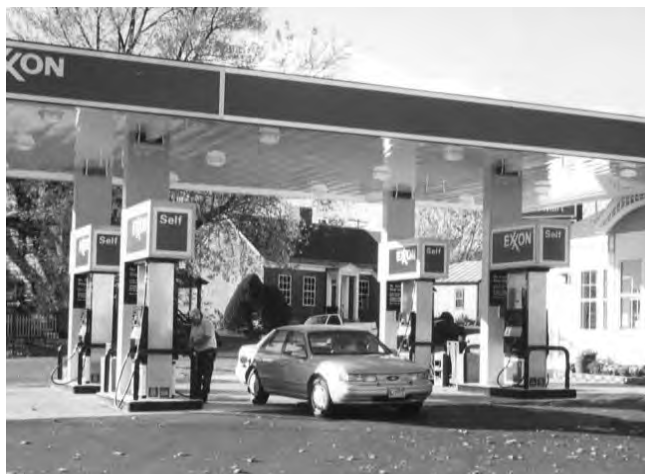
Drop fixtures are not allowed since they can produce dangerous levels of glare and cause a nuisance to abutting properties.
