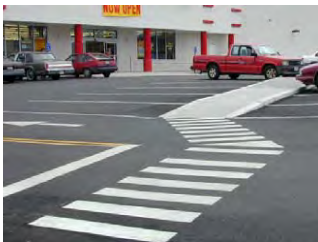
A raised walkway that provides a high level of contrast with the surrounding parking lot. However, the width of the walk is compromised by the overhang of the cars, making pedestrian movement difficult.
