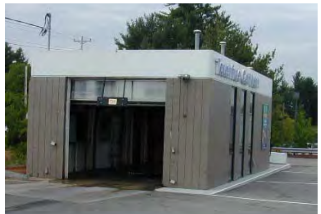
An accessory structure (a freestanding car-wash) that would not meet the design guidelines for form and materials.
