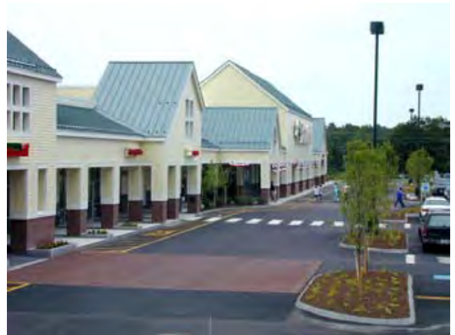
These wide parking lot islands will provide ample room for tree growth.
