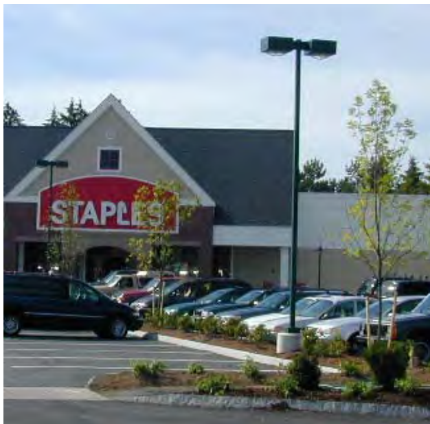
These light fixtures have been coordinated with the planting plan to avoid problems as the trees mature. Slightly raised bases protect the poles from plow damage.
