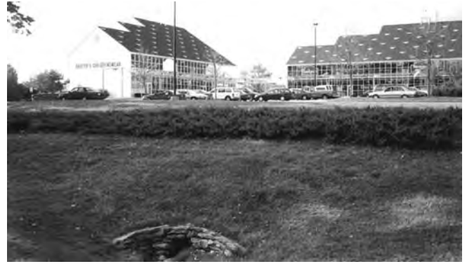
Motorists driving past this shopping center only see the low juniper hedge, unaware of the detention basin on the far side. Hand-placed stonework protects the end of the culvert.
