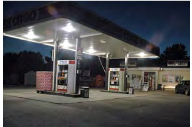
An example of dropped canopy fixture that spills light beyond the property line and causes potentially hazardous glare.
