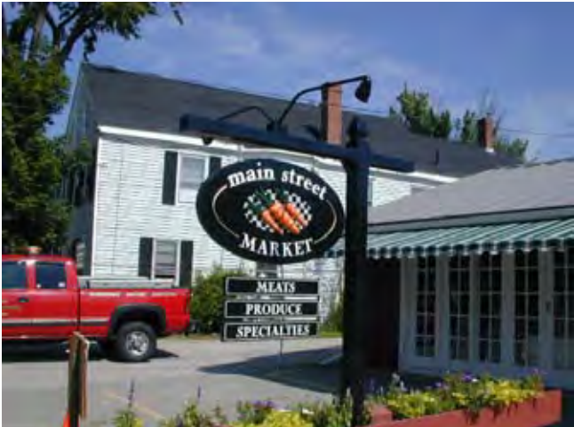
Small spotlights directed downward are easily aimed to prevent glare. The simple design of the fixture complements the line and colors of the sign.
