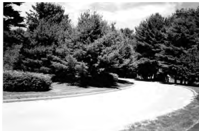
A 6-8' high earth berm, planted with evergreen trees and shrubs, creates an effective screen to separate an access drive from residential properties.
