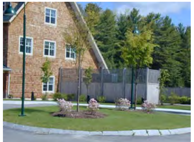
Mechanical units for senior housing are hidden behind a fence with opaque and translucent panels.
