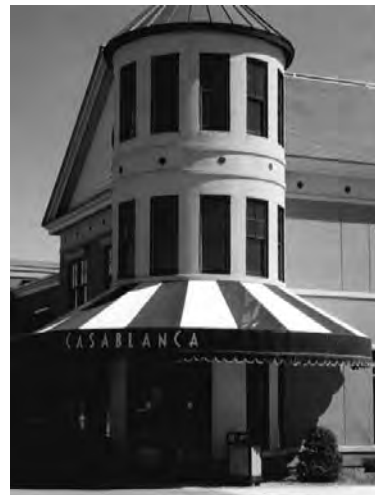
Canopies over doorways can emphasize the main entrance and provide effective protection from the elements. The name of the theater is incorporated into canopy and counted toward the total signage area.
