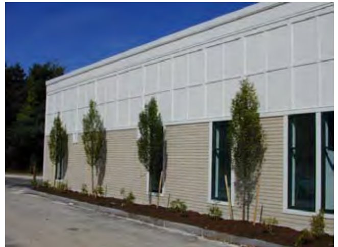
Upright forms of tree species were selected for this tight location next to a building wall.
