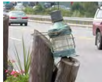
Low pedestrian lights must be well constructed and secured to a permanent base to prevent damage and dislocation. The fixture on the left appears unstable and prone to damage. The bollards on the right provide even illumination and complement the building.
