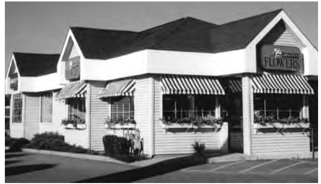
Awnings can be used effectively to add scale, visual interest and provide shade to the building facade.
