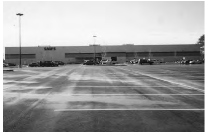
Landscaped islands should have been used here to provide scale, reinforce internal circulation routes, and lead pedestrians to the entrance.
