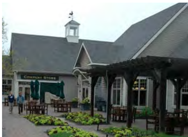
The cupola projecting from this pitched roof is an example of traditional forms used in a contemporary structure.
