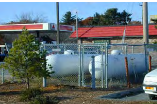
Chain link fence provides security, but is too transparent to provide any visual screening.
