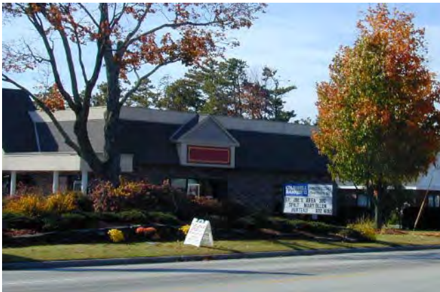
New development with parking on the side, extensive landscaping, preserved trees, and building relatively near the street,
