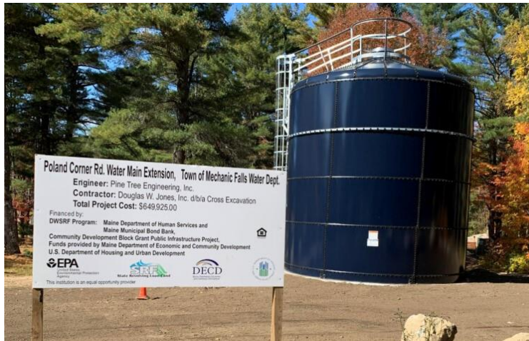
Poland Corner Road Water Tank Shortly After Construction
