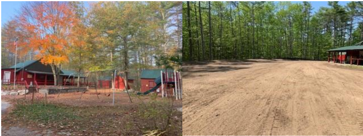
Camp Connor Main Building Front and Rear View (the berm has just been removed)
