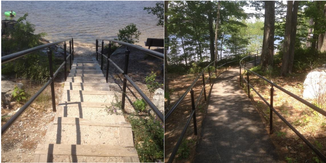
Tripp Lake Beach – Stair and Ramp Access
