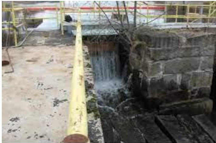
Thompson Lake Dam
