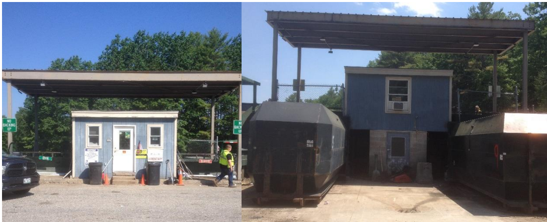
Transfer Station Main Office and Trash Disposal Area – Front and Rear View
