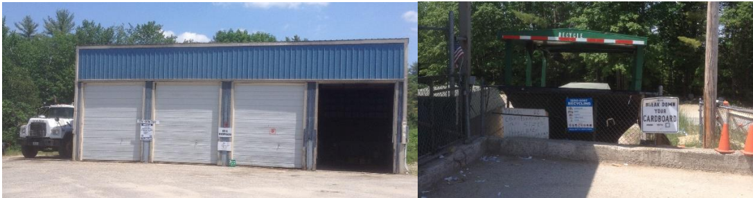
Recycling Garage – Waste Oil and Electronic Waste, and Single Sort Recycling
