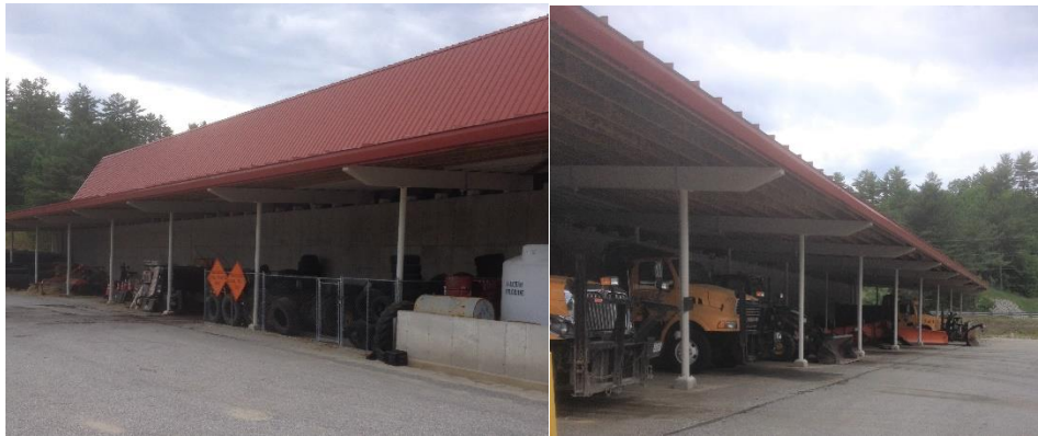
Salt Barn Equipment and Vehicle Storage
