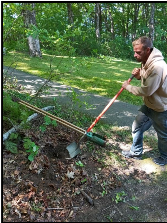
Josh Harlow preparing installation of one of the 14 panels
