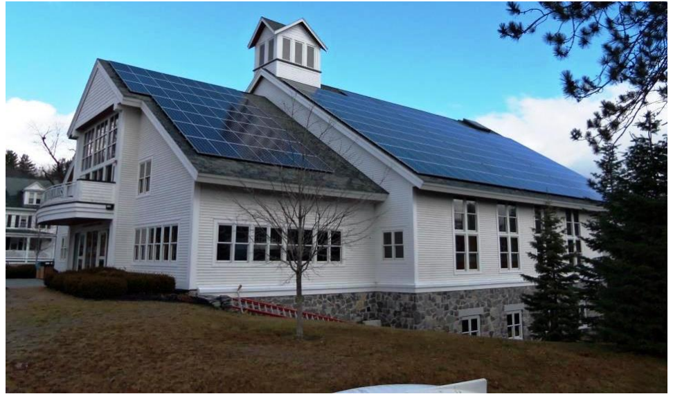
74 kilowatt PPA project at Proctor Academy in Andover, NH
