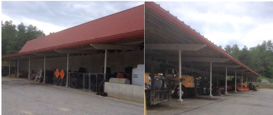
Salt Barn Equipment and Vehicle Storage
