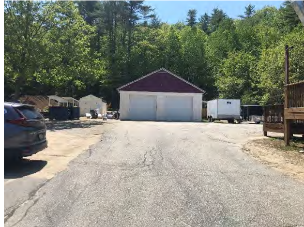
Old Fire Station/Recreation
