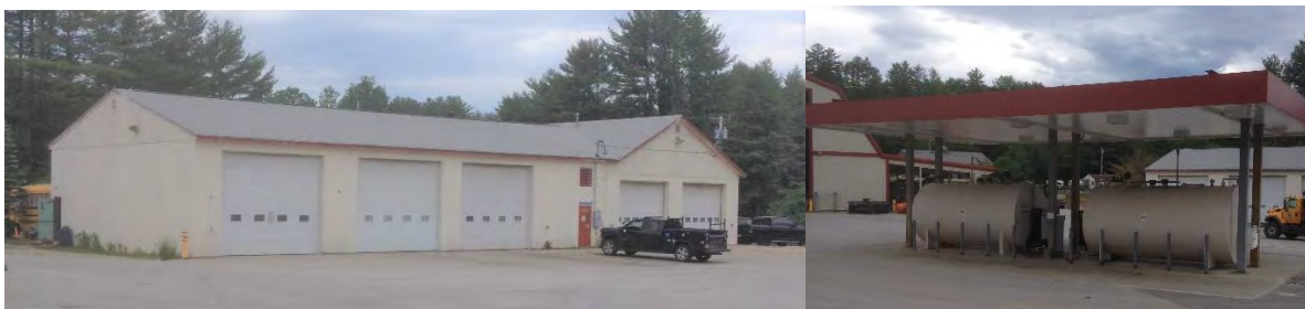
Poland Public Works Garage and Office, and Fuel Tanks and Pumps
