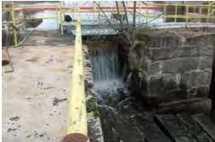
Thompson Lake Dam
