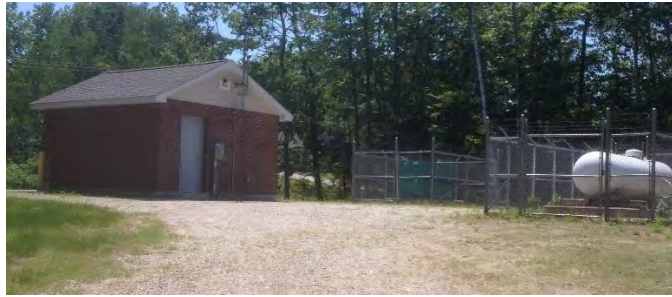
Sewer Pump Stations on RT 122
