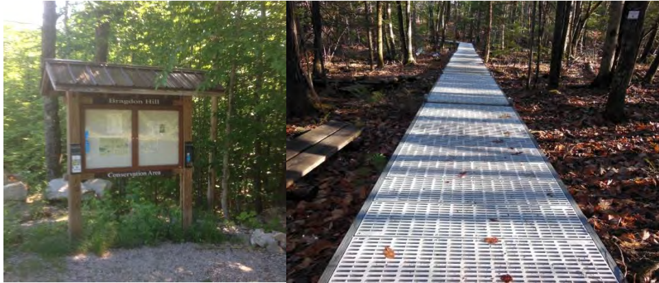
Bragdon Hill Trail Head and Trail Bridge Section
