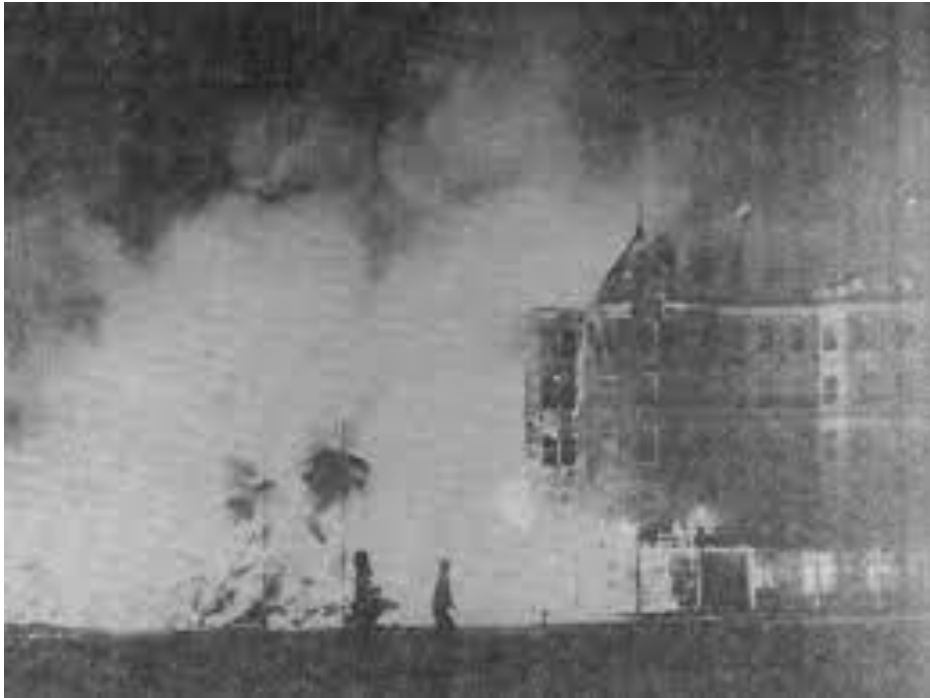
Poland Spring House Fire
