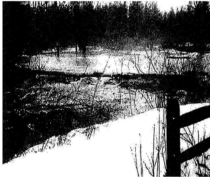
Flooded Roadway Turkey Lane Road Livermore, ME April 2005
