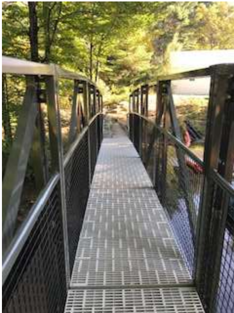
Waterhouse Brook Dam Bridge
