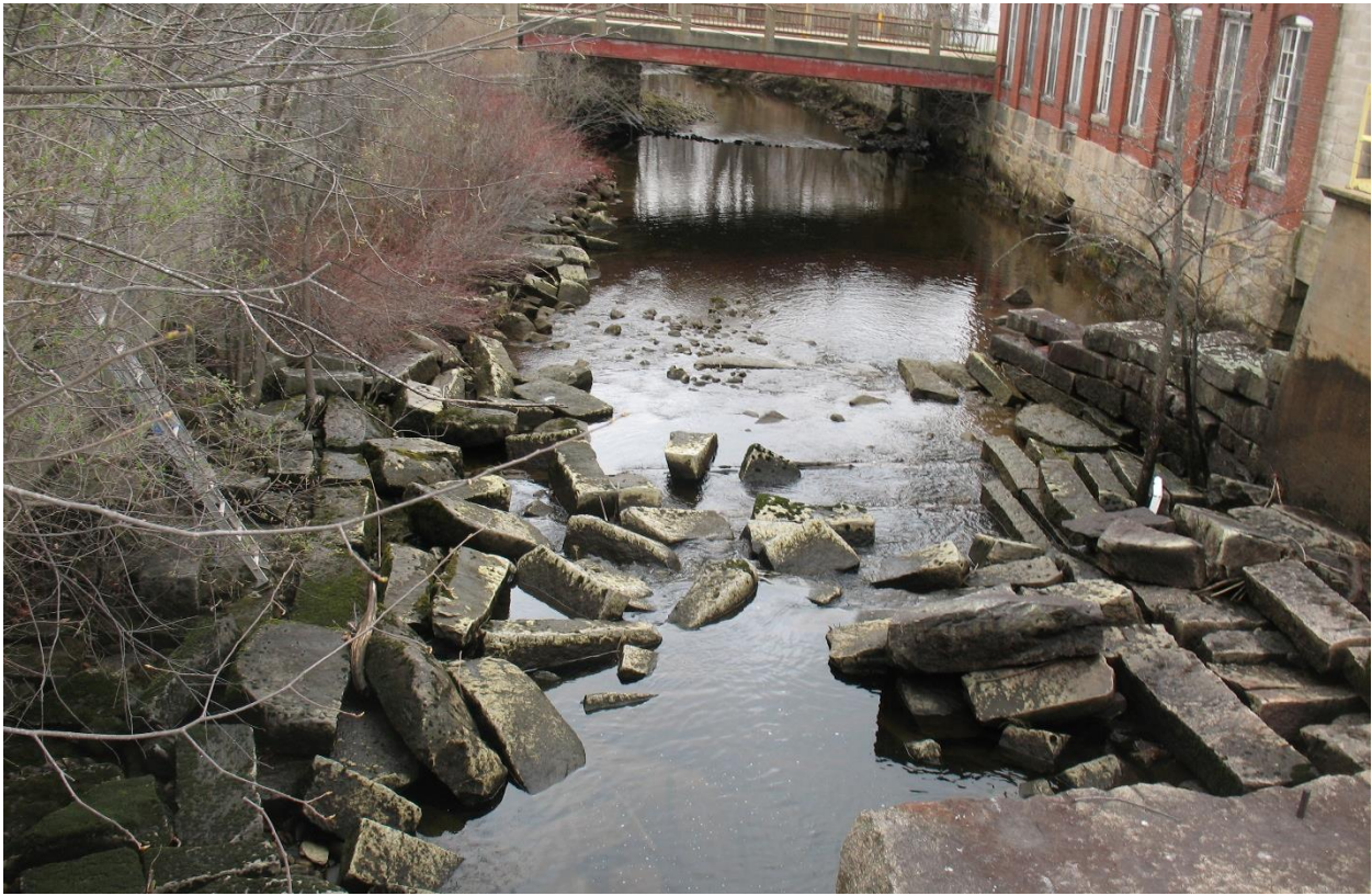
Photo 6. Downstream Channel from Top of Dam, 5/4/2018
