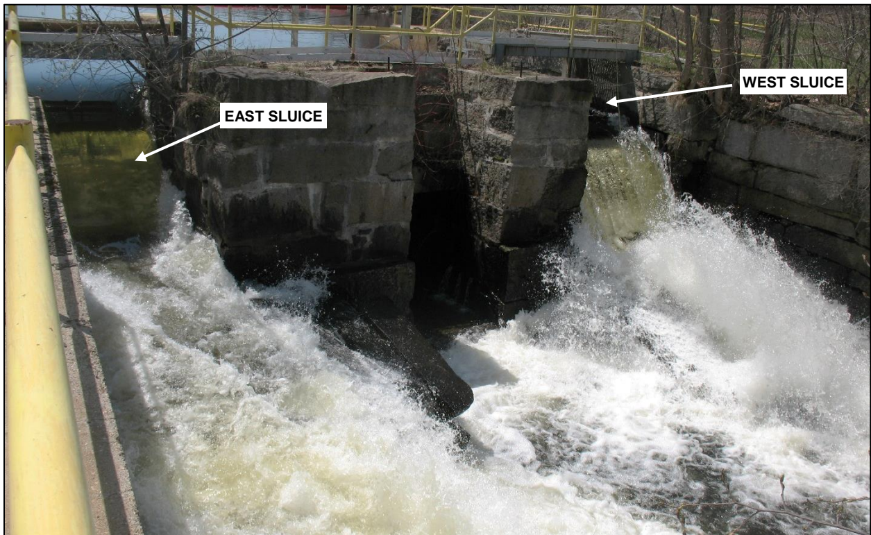
Photo 9. Downstream View of Dam with East and West Sluice Stoplogs Removed, 5/2/2018
