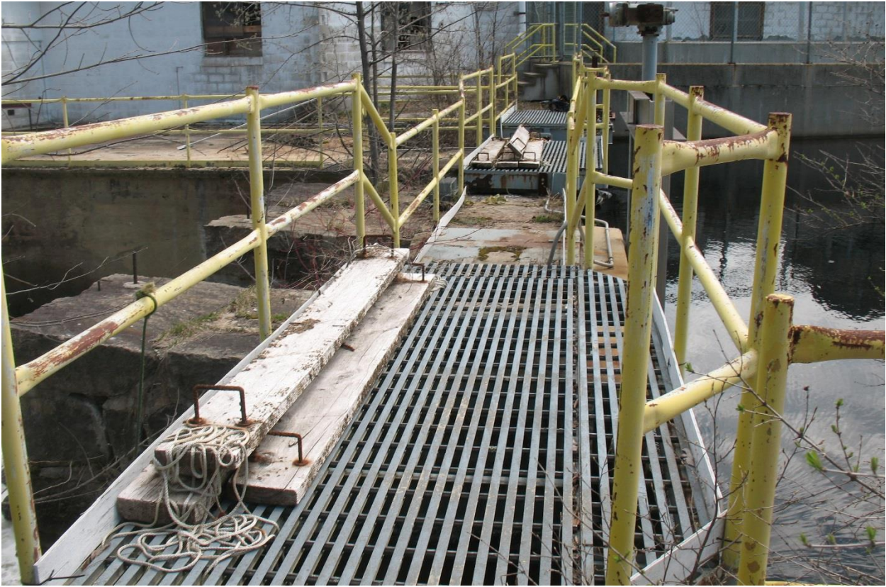
Photo 4. Top of Dam from West Abutment, 5/2/2018
