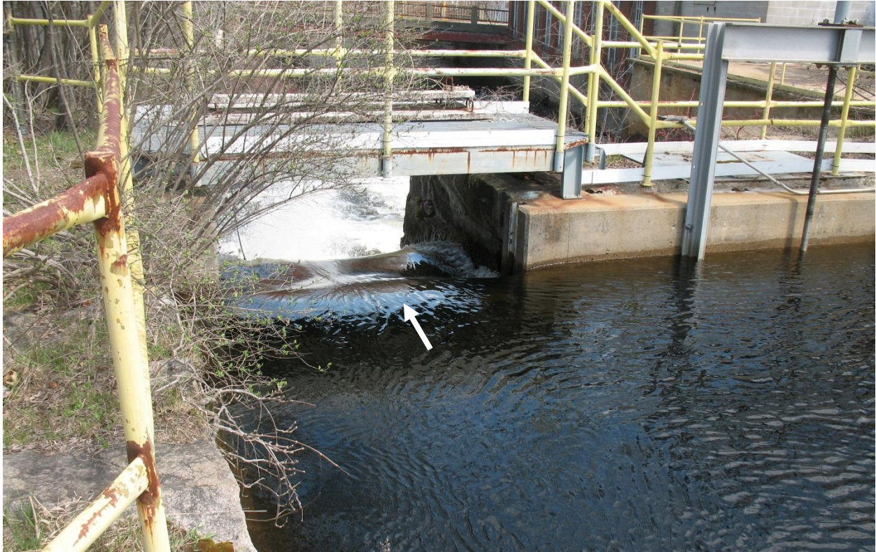
Photo 8. Upstream View of Discharging West Sluice (arrow), 5/2/2018
