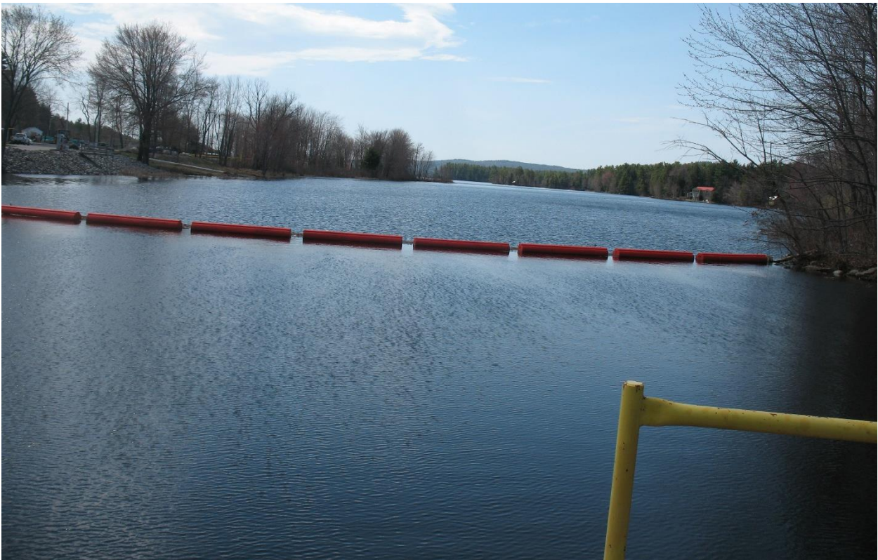
Photo 5. Thompson Lake from Top of Dam, 5/2/2018
