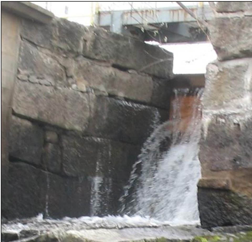
Photo 15. East Sluice Left Wall: Open Voids and Leakage in Masonry.
