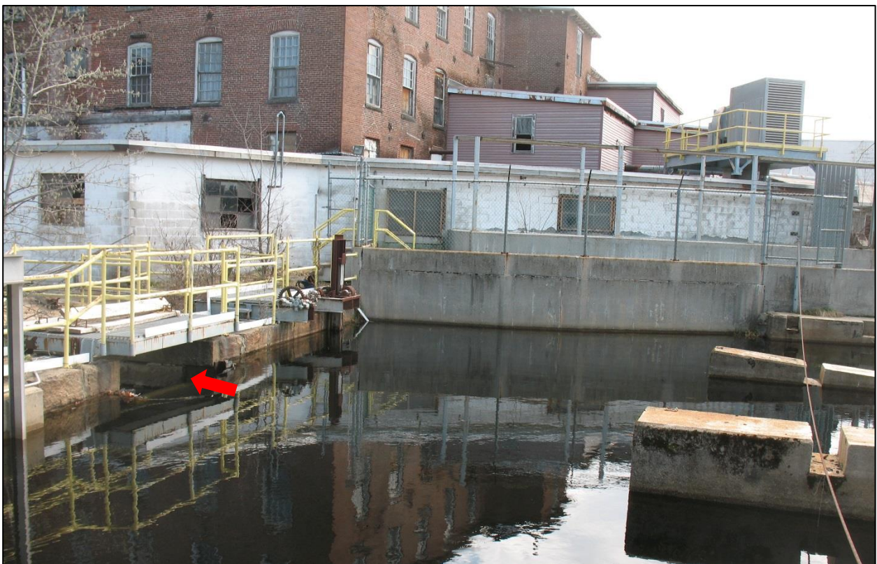
Photo 12. Upstream View of East Sluice.
