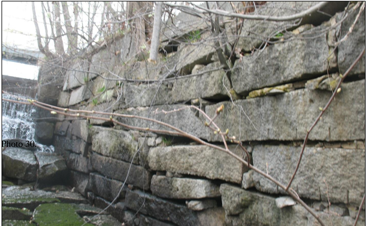
Photo 29. View of Left Discharge Channel Retaining Wall from Dam. Note Bulging, Displaced and Missing Stone, Voids, Large Trees and Brush.
