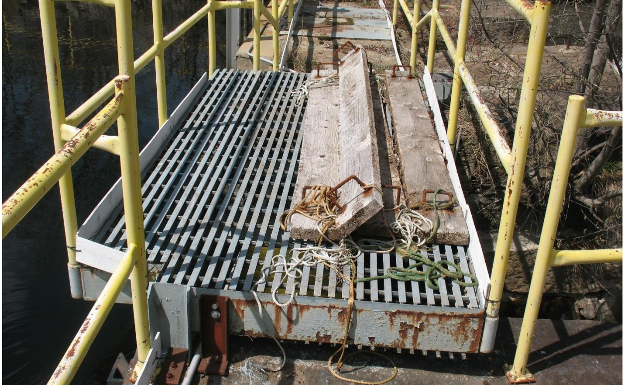
Photo 10. Upper East Sluice Stoplogs Removed to Pass Flow, 5/2/2018
