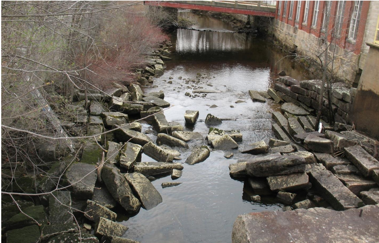
Photo 25. Discharge Channel. Left Channel Side Obscured by Dense Vegetation.
