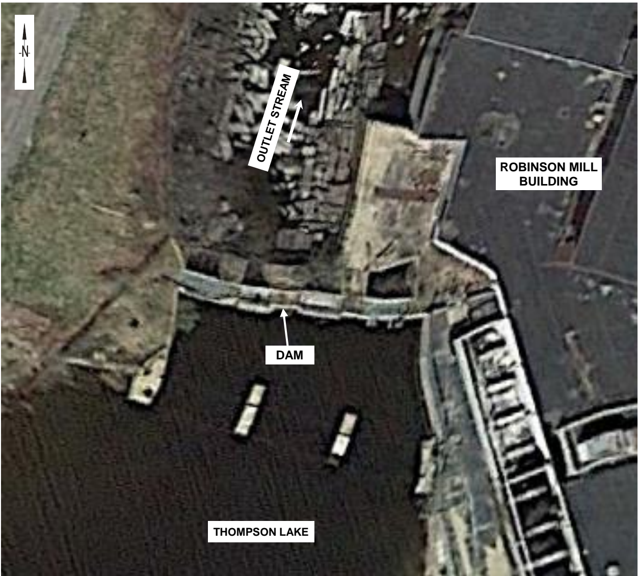
Photo 1. Aerial View of Dam Site. Google Earth, 2018
