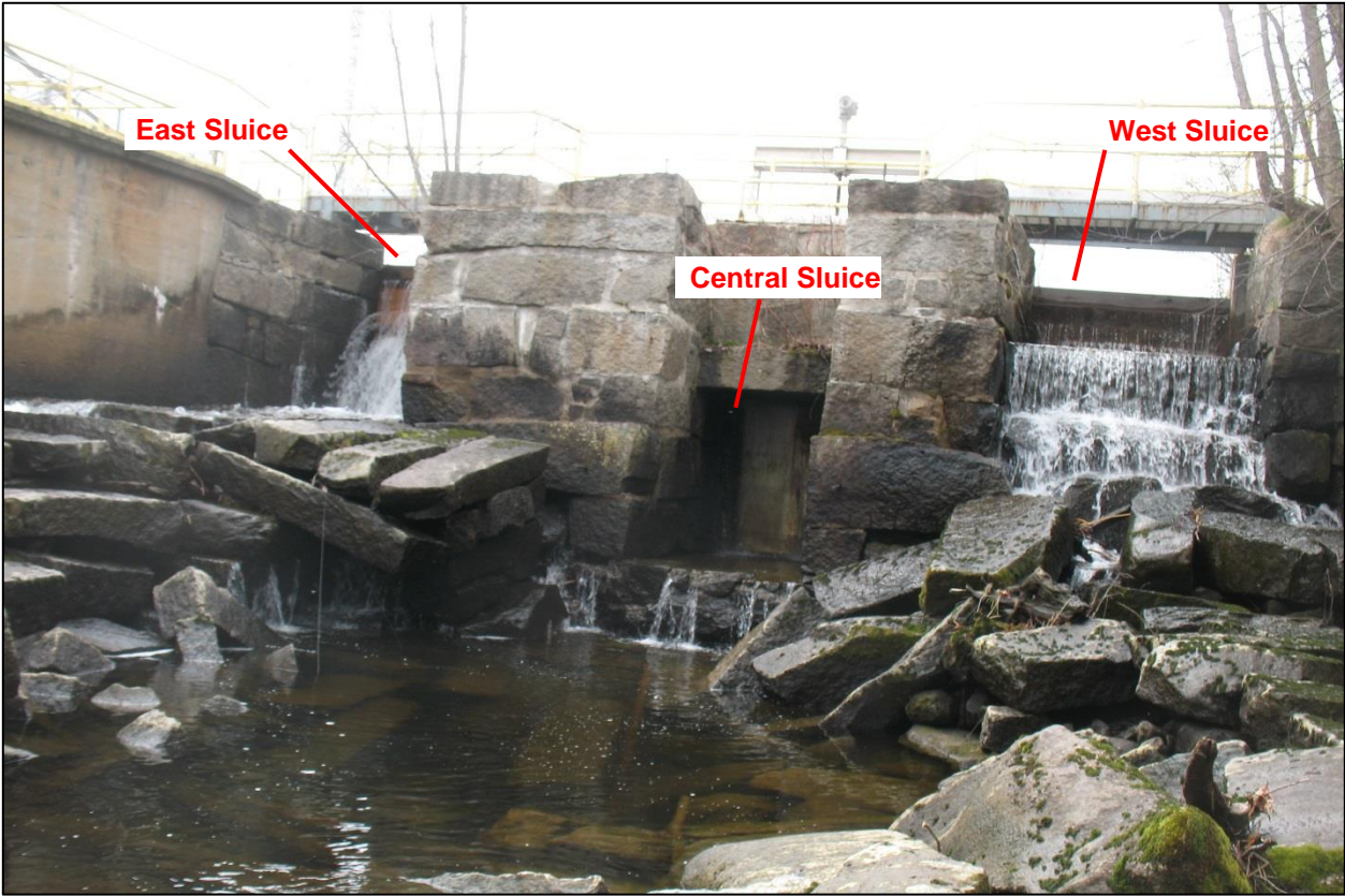
Photo 2. Downstream View of Dam.
