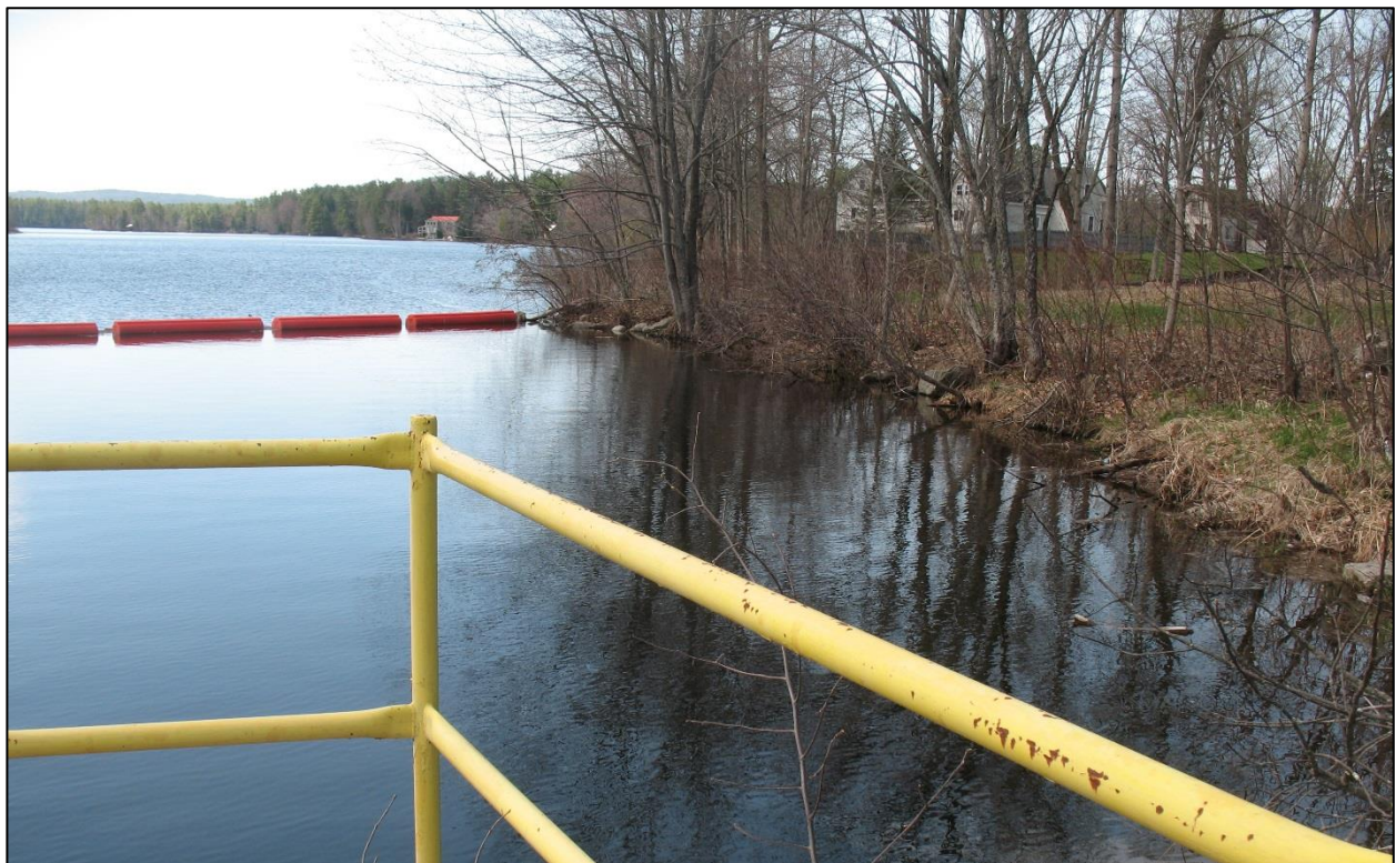
Photo 22. Left Approach Channel Bank Between Log Boom and Dam. Note Large Trees at Waterline.
