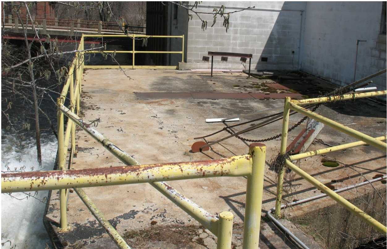
Photo 20. Downstream View of Concrete Dam Section.
