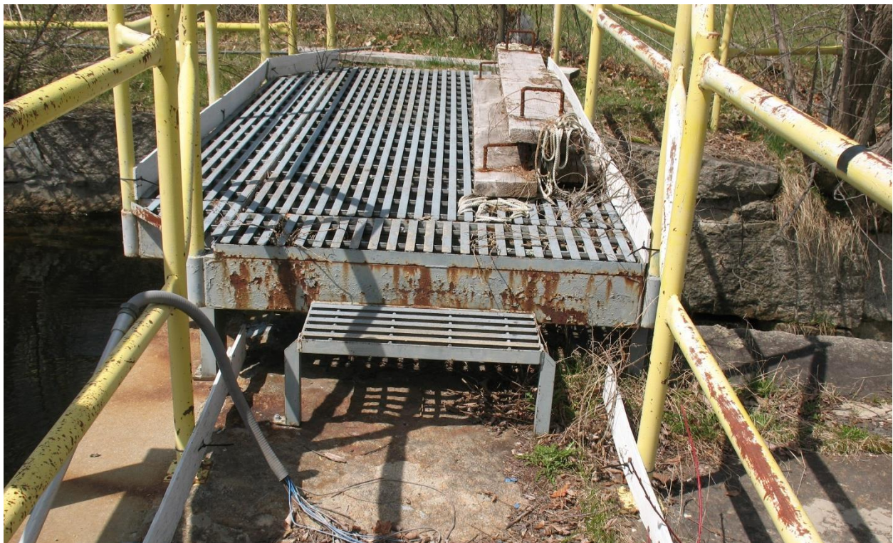
Photo 6. West Sluice Operating Platform.
