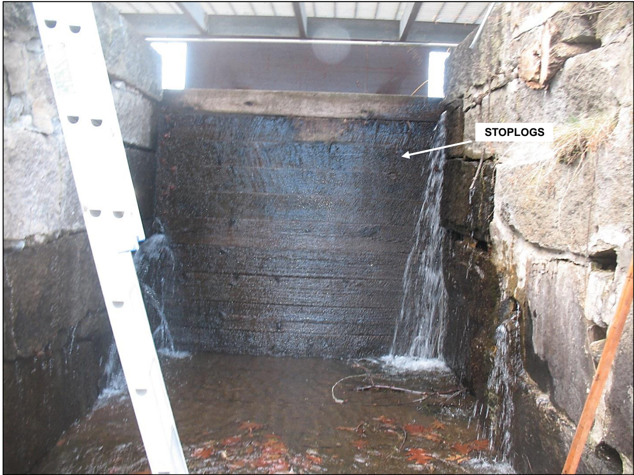
Photo 12. Downstream View of East Sluice Stoplogs and Masonry Walls, 12/4/2018
