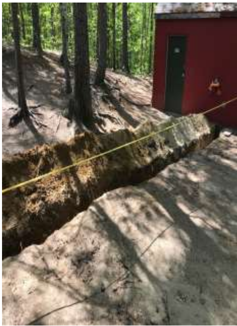
Ditching for electrical work to install hot water heaters
