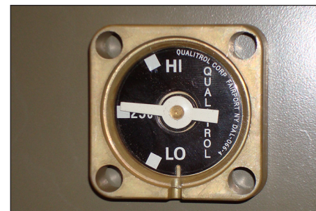
Figure 6. Liquid level gauge.
