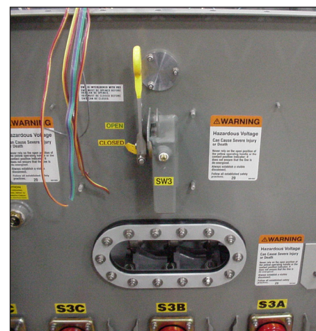
Figure 7. VFI transformer with visible break.
