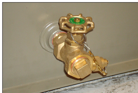
Figure 4. Drain valve with sampler.
