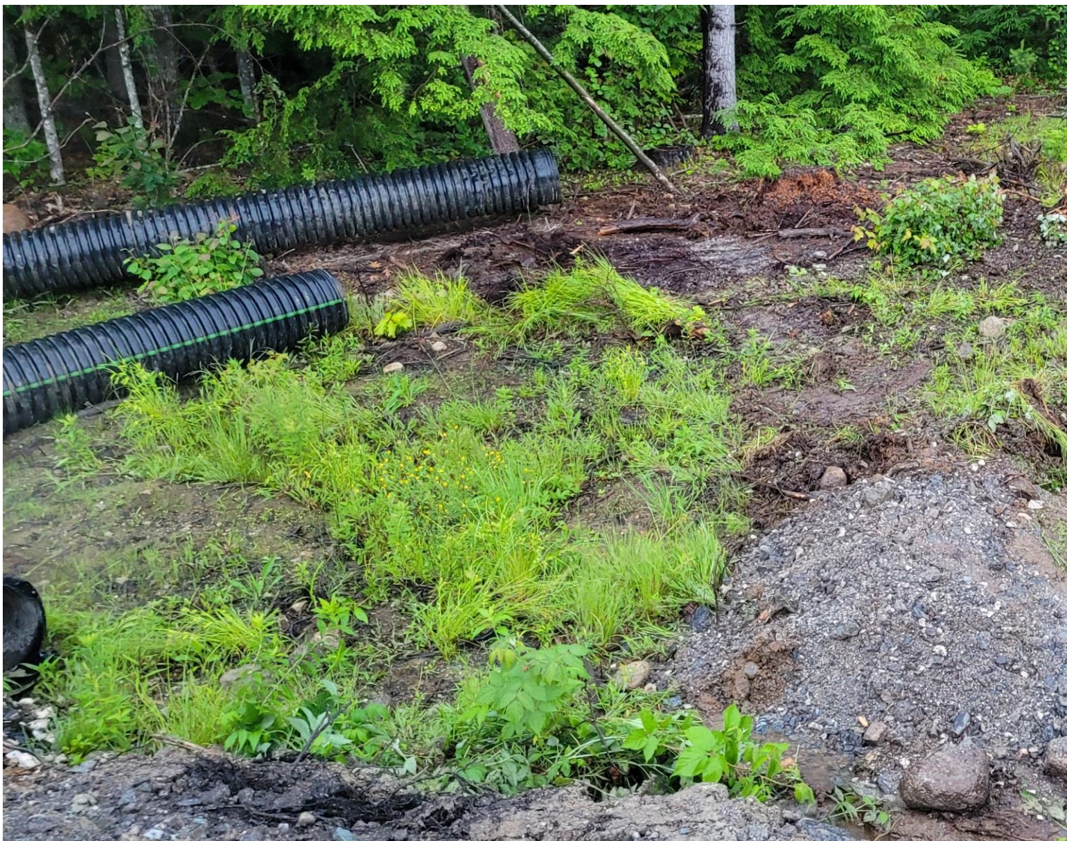
Edge of current road terminus with culvert projecting from the sideslope. Pipe should be cut back and areas protected with erosion control, or stone lined, until revegetated.
