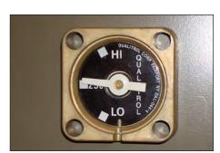
Figure 6. Liquid level gauge.
