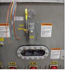
Figure 7. VFI transformer with visible break.
