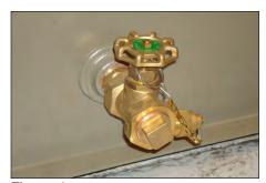
Figure 4. Drain valve with sampler.
